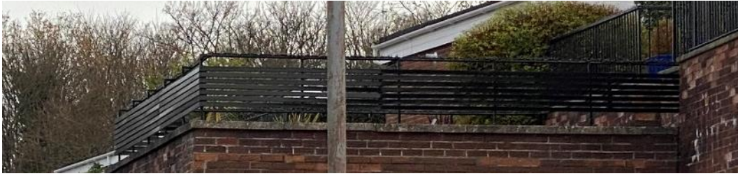
Open bar fencing on Dunvegan Avenue
